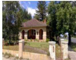
Former UV Knight's House, 26 Ogilvy St
