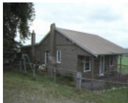
yeringberg maroondah hwy coldstream cottage view dec1987
