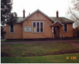
Nyora Railway Station complex
