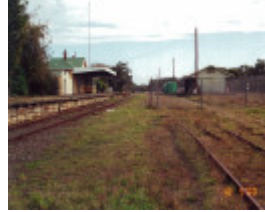
Nyora Railway Station complex
