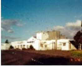
Former Poowong Butter Factory (2000)
