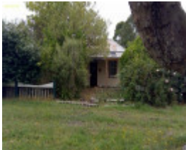
Butter Factory Manager's Residence (former, 2020)
