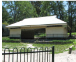
AUBURN PRIMARY SCHOOL NO.2948 SOHE 2008
