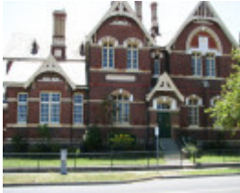
AUBURN PRIMARY SCHOOL NO.2948 SOHE 2008
