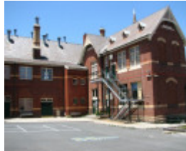
AUBURN PRIMARY SCHOOL NO.2948 SOHE 2008
