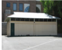
AUBURN PRIMARY SCHOOL NO.2948 SOHE 2008
