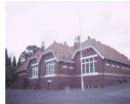
auburn primary school no 2948 rear view
