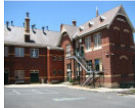
AUBURN PRIMARY SCHOOL NO.2948 SOHE 2008
