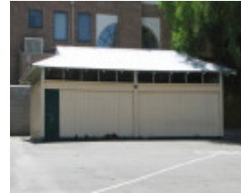
AUBURN PRIMARY SCHOOL NO.2948 SOHE 2008
