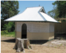
AUBURN PRIMARY SCHOOL NO.2948 SOHE 2008
