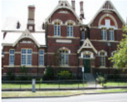
AUBURN PRIMARY SCHOOL NO.2948 SOHE 2008
