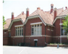
AUBURN PRIMARY SCHOOL NO.2948 SOHE 2008
