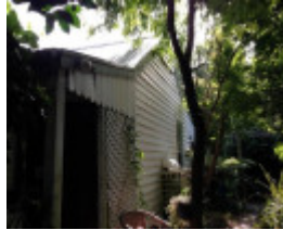
South side elevation of north cottage
