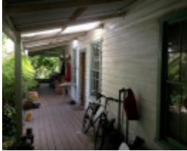
Looking to the north along verandah of north cottage
