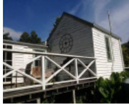
Formerly detached rear kitchen (now bathroom)
