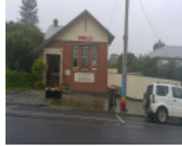
Toora Post Office
