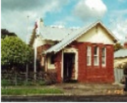
Toora Post Office (2000)
