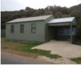
Walkerville North Public Hall
