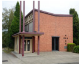
All Saints (former Christ Church) Mitcham, detail of entrance, 2012.JPG
