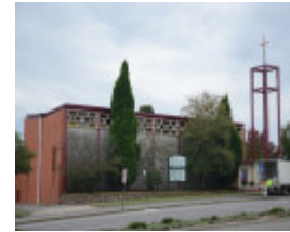
All Saints (former Christ Church) Mitcham, south elevation, 2012.JPG
