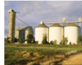
1 former wimmera flour mill & silo complex gibson street rupanyup silos side view
