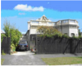
48 Stanhope Street Malvern
