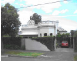
54 Stanhope Street Malvern
