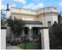
86 Stanhope Street Malvern
