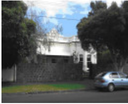
88 Stanhope Street Malvern
