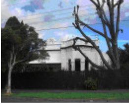
92 Stanhope Street Malvern
