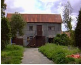
WORKSHOP AND STABLES (FORMER)
