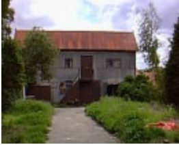
WORKSHOP AND STABLES (FORMER)
