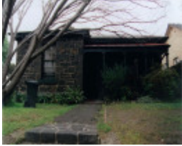
POLICE HEADQUARTERS (FORMER)
