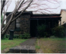
POLICE HEADQUARTERS (FORMER)
