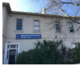
1219-1225 Dandenong Road, Malvern East
