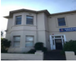
1219-1225 Dandenong Road, Malvern East
