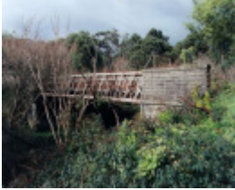
OLD LOWER PLENTY BRIDGE
