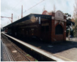
HEIDELBERG RAILWAY STATION
