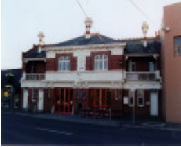
IVANHOE METROPOLITAN FIRE BRIGADE STATION
