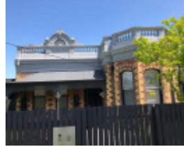
50 Stanhope Street, Malvern
