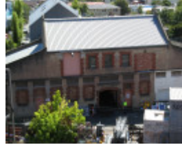
Municipal stables Sth Yarra_south side_18 Feb 08
