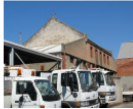
Municipal stables Sth Yarra_north side_18 Feb 08
