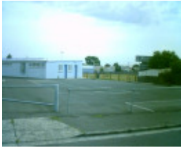
90-100 Shannon Avenue, Geelong West - Reserve
