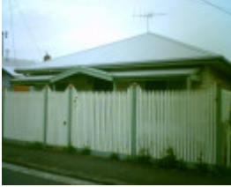
74 Waratah Street, Geelong West
