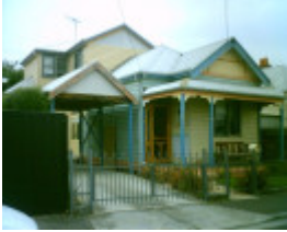
79 Waratah Street, Geelong West
