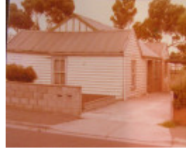
Source GRS1160 Geelong Heritage Centre, c1981-85
