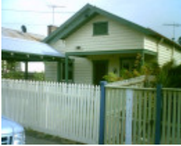
90 Waratah Street, Geelong West
