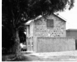
Carlisle Stables, now 10 Bannerman Street, Bendigo
