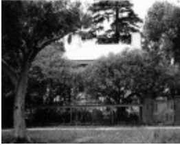
Carlisle House, 12 Bannerman Street, Bendigo
