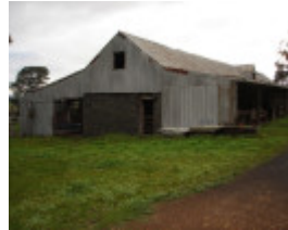
Summer Hill large cow shed from south KJ 10 July 07 69
