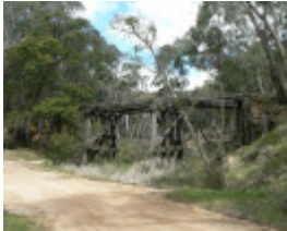
Mt Misery Creek Trestle Bridge, Berringa
