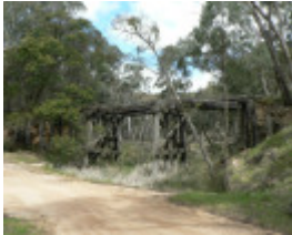
Mt Misery Creek Trestle Bridge, Berringa
