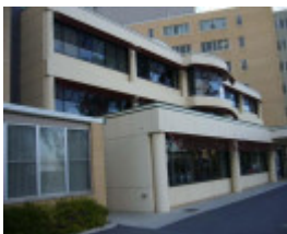
John Lindell Rehabilitation Unit 1999
