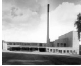
Boiler House and Laundry 1956
