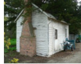
Linton Park Linton Mannibadar Rd Linton, laundry at rear.
