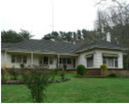
Linton Park Linton Mannibadar Rd Linton, viewed from the north-east
