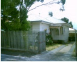
20 Catherine Street, Geelong West
