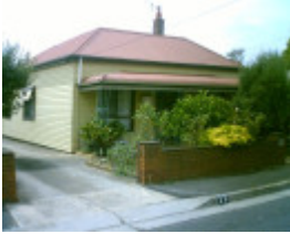
22 Catherine Street, Geelong West
