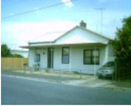
27 Catherine Street, Geelong West
