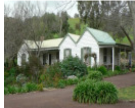
Former Mill Managers Residence
