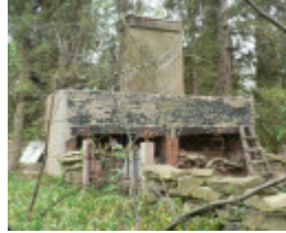
31709 Lawson's Hotel Cambridge St former kitchen chimney 374
