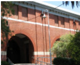
AUBURN RAILWAY STATION COMPLEX SOHE 2008
