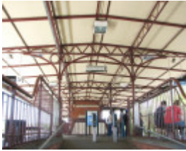
AUBURN RAILWAY STATION COMPLEX SOHE 2008
