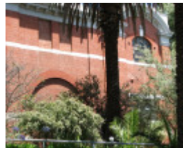
AUBURN RAILWAY STATION COMPLEX SOHE 2008
