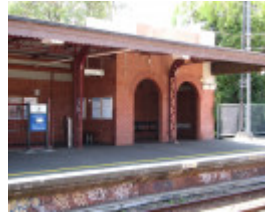
AUBURN RAILWAY STATION COMPLEX SOHE 2008
