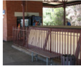
AUBURN RAILWAY STATION COMPLEX SOHE 2008
