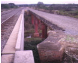
rail bridge creswick creek top view may1995
