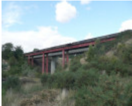
RAIL BRIDGE SOHE 2008
