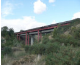
RAIL BRIDGE SOHE 2008
