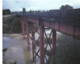
1 rail bridge creswick creek side view may1995
