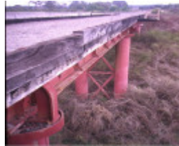
rail bridge creswick creek siding detail may1995
