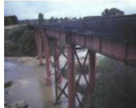
1 rail bridge creswick creek side view may1995
