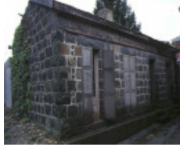
1 former creswick gold office front view
