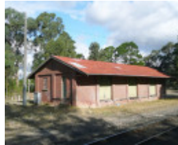
CRESWICK RAILWAY STATION COMPLEX SOHE 2008
