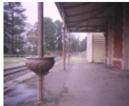
creswick railway complex platform may1995
