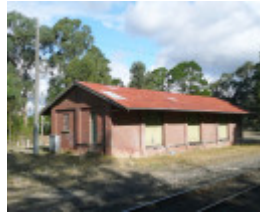
CRESWICK RAILWAY STATION COMPLEX SOHE 2008
