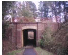
creswick railway complex pedestrian subway may1995
