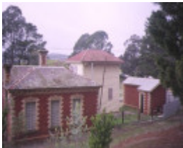
creswick railway complex rear view may1995
