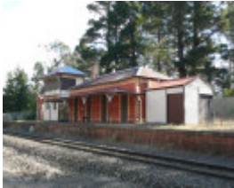
CRESWICK RAILWAY STATION COMPLEX SOHE 2008
