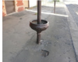
CRESWICK RAILWAY STATION COMPLEX SOHE 2008
