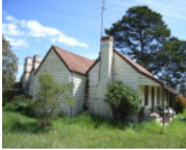
204539 11 Argyle Road, Argyle
