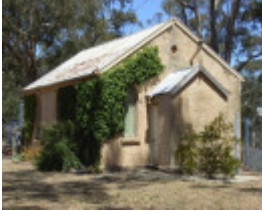
Wesleyan Church (former), 204623 1 McClellans Crescent, Argyle
