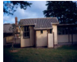
H02030 point nepean isolation hospital
