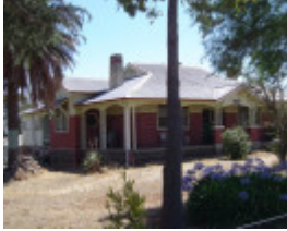
215715 381 Axedale Kimbolton Road, Axedale
