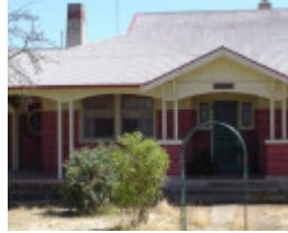
215715_Axedale_Axedale Kimbolton Road_381_img03
