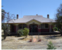
215715_Axedale_Axedale Kimbolton Road_381_img02
