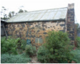
Outbuilding, 358 Brownes Lane, Axedale
