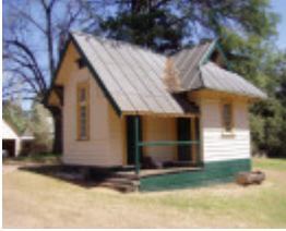
2270 Mclvor Highway, Axedale Marydale outbuildings
