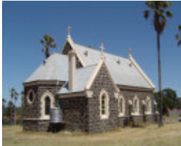
15 Raglan Place East, Axedale. St Mary's Catholic Church
